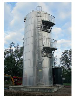
One HydroSystemTower<sup>®</sup> with a volume of 2 x 30 m<sup>3</sup>, an integrated pressure booster system, extensive installation and a control system was manufactured, moved to its installation site and commissioned to supply water to a military training area in eastern Germany.
