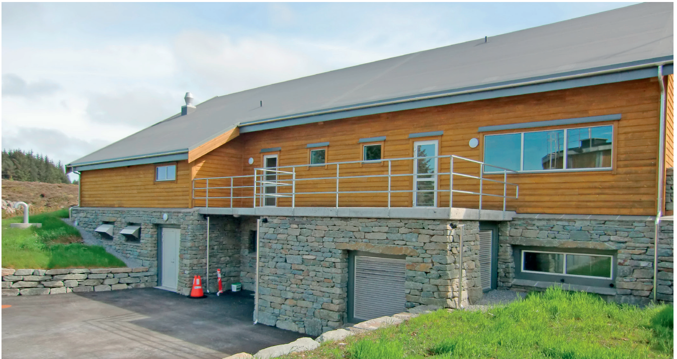
Overview (Source: Hydro-Elektrik GmbH)
